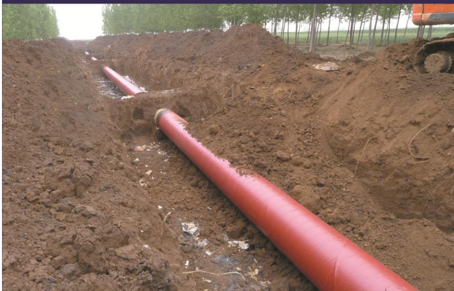
Rehabilitation of Existing Pipeline ▲
